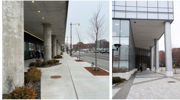
Figures | (Left) Sidewalk along the Lydian on Damen Avenue; Sidewalk along Polk Street at Rush
