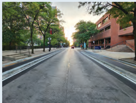
FIGURE 6: POLK STREET PROTECTED BIKE LANES
