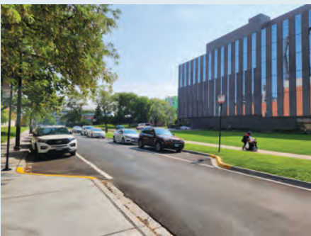
FIGURE 5: HERMITAGE AVENUE RESURFACING
